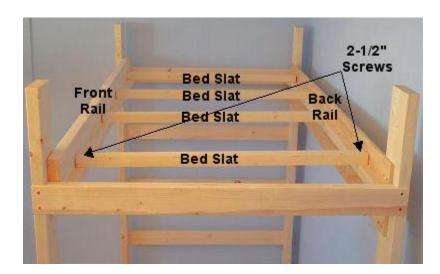
Insert the bed slats between the front and back rails, evenly spacing them apart. You can now completely tighten the carriage bolts. Fasten the bed slats to the front and back rails using 2-1/2 In. screws.
