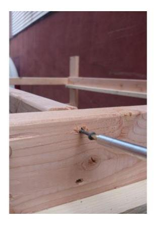
Allign the two front rails in a perpendicular fashion. Screw (2) 2-1/2 Coarse Screws in the pre-drilled hole to connect the two beds.
