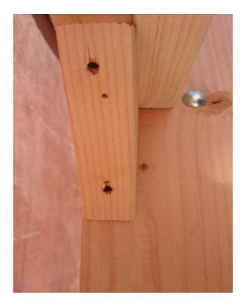
Install the Angle Bracket under the back rail on your wall side. Use the 2-1/2 In. Coarse Screws to mount it under the back rail and post.
