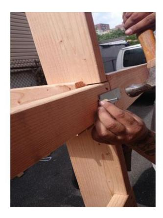
Use the Metal Nail Stopper connect the two back rails together as shown. Use the two 1-1/2 In. Galvanized Nails provided.
