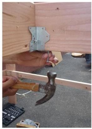
Start to connect the two seperate beds, you have just made, using the Metal Angle Bracker. Hammer the 12 1-1/2 In. Galvanized Nails through the holes in the metal.
