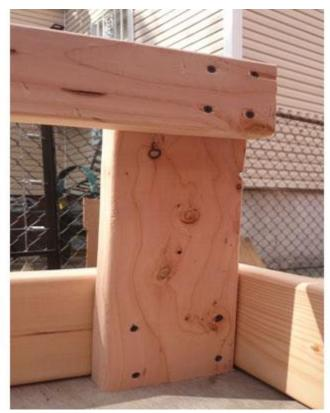
Install the Safety Rails Support Bar on top of the Metal Angle Bracket. This will support the Youth Safety Rail. Use 2-1/2 In. Coarse Screws to attach the support to the Front Rail and Safety Rail. Screw with 2-1/2 In. Coarse Screws from the perpendicular Safety Rail to this support as well.
