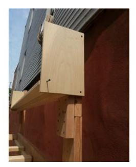
Screw the side pieces  $(3/4" \times 8-1/2" \times 12-3/4" \text{ Ply})$  with 1-5/8" Black Course Screws into the side of the Ply Shelf installed in above step.
