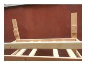
Attach 2 Bookshelf post (2 x 6 x 18") to the Top of the Back Legs With 2-1/2" Black Course Screws. Connect with Two post connectors  $2 \times 6$ .
