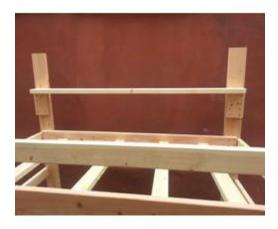
Place the Shelf Support  $(2 \times 4)$  flat on top of the Bookcase post and screw on tight with 2-1/2" Black Course Screws into the new post extension support installed in step above.
