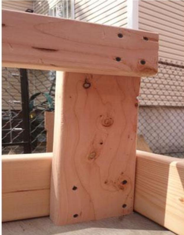
Install the Safety Rails Support Bar on top of the Metal Angle Bracket. This will support the Youth Safety Rail. Use 2-1/2 In. Coarse Screws to attach the support to the Front Rail and Safety Rail. Screw with 2-1/2 In. Coarse Screws from the perpendicular Safety Rail to this support as well.
