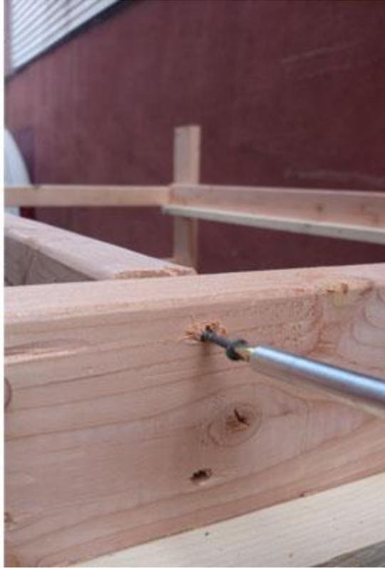
Align the two front rails in a perpendicular fashion. Screw (2) 2-1/2 Coarse Screws in the pre-drilled hole to connect the two beds.
